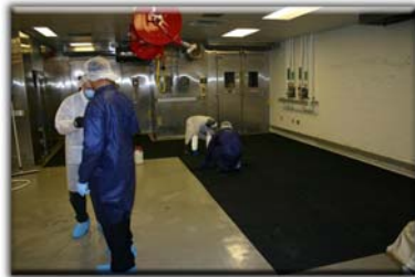
Fiberglass Floor Installation
