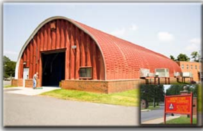
Quonset Hut Structure
