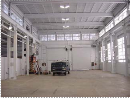
This project converts an empty warehouse into usable office space.
