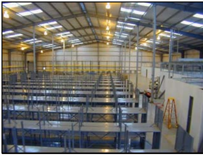
Phase I: Overview of Shelving, 1 st level
