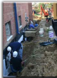
Waterproofing for Research Lab
