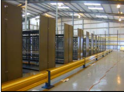
Phase I: Shelving & Aisle Guard
