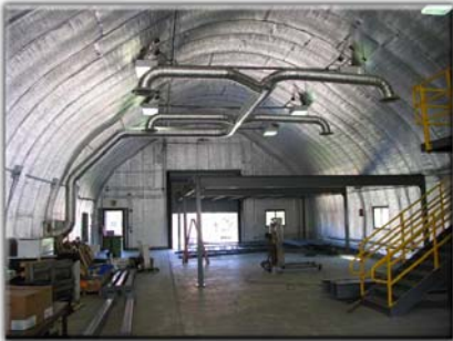
Inside Structure...Before Construction
