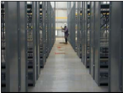
Phase I: Phase I installation nearing completion
