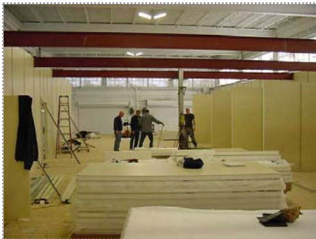
Initial installation of two-level office space & catwalk.
